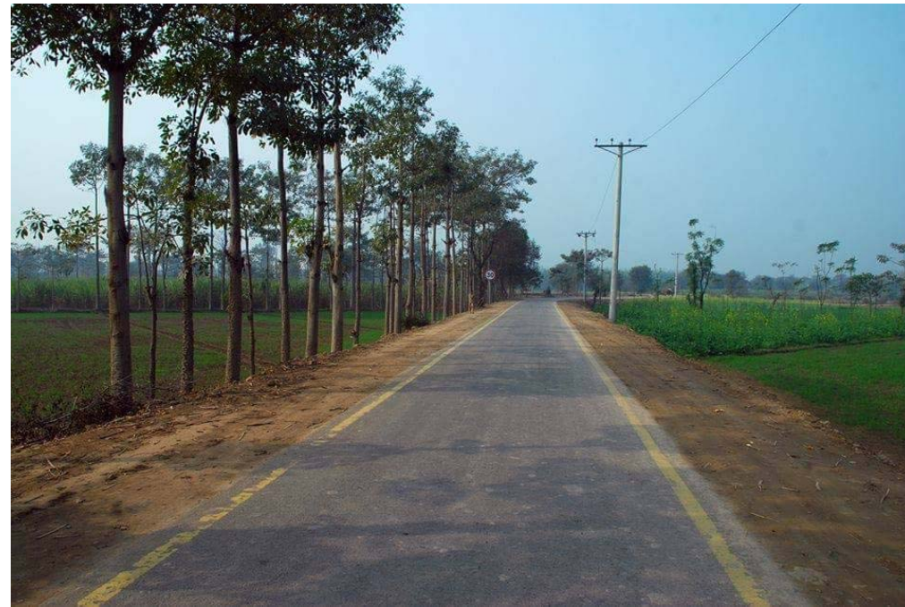
Rural road and electricity in Kasur District, Punjab Province, Pakistan
