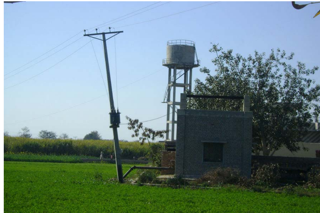
Rural electricity and drinking water facilities in Kasur District, Punjab Province, Pakistan.
